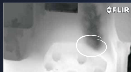
CAPTURED GAS LEAK
