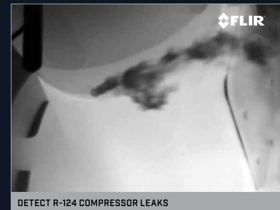
DETECT R-124 COMPRESSOR LEAKS
