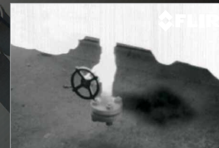
METHANE LEAK AT NATURAL GAS FACILITY SITE
