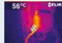
What a thermal imaging camera sees.
