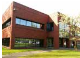
FLIR Systems, Portland
