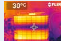
What a thermal imaging camera sees.
